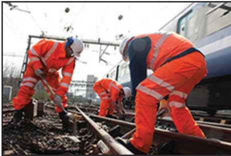
Image 41. Railway infrastructure, track repair crew.
