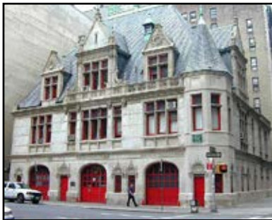
Democracy Now! In Exile Old Firehouse operated by DCTV Attic Studio — tiny, drafty and safe
